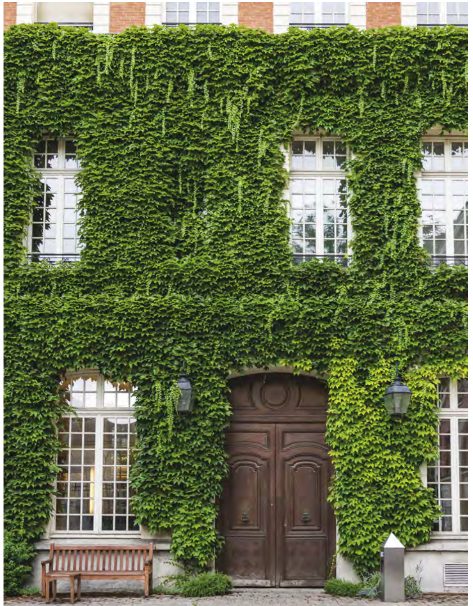
Charming architecture characterises the Marais, from confectioner Méert's shopfront (opposite) to the ivy-covered Hôtel Duret de Chevry (above)
